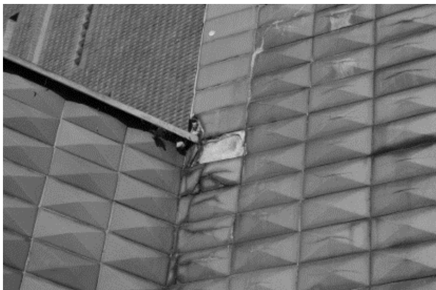
Figure 2. The degradation processes affect especially the cusps of the tiles. The cracking of the glaze evolves in the fracture of the ceramic body with loss of tiles. It is possible to recognize the efflorescences along the path of flow of water.
